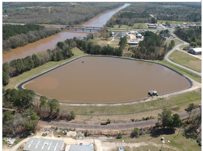
Harnett Regional Water – Water Treatment Plant Reservoir
